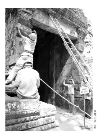
**Photo 1.** WMF Khmer architect and draftsmen preparing for structural consolidation of western gate, Preah Khan.
