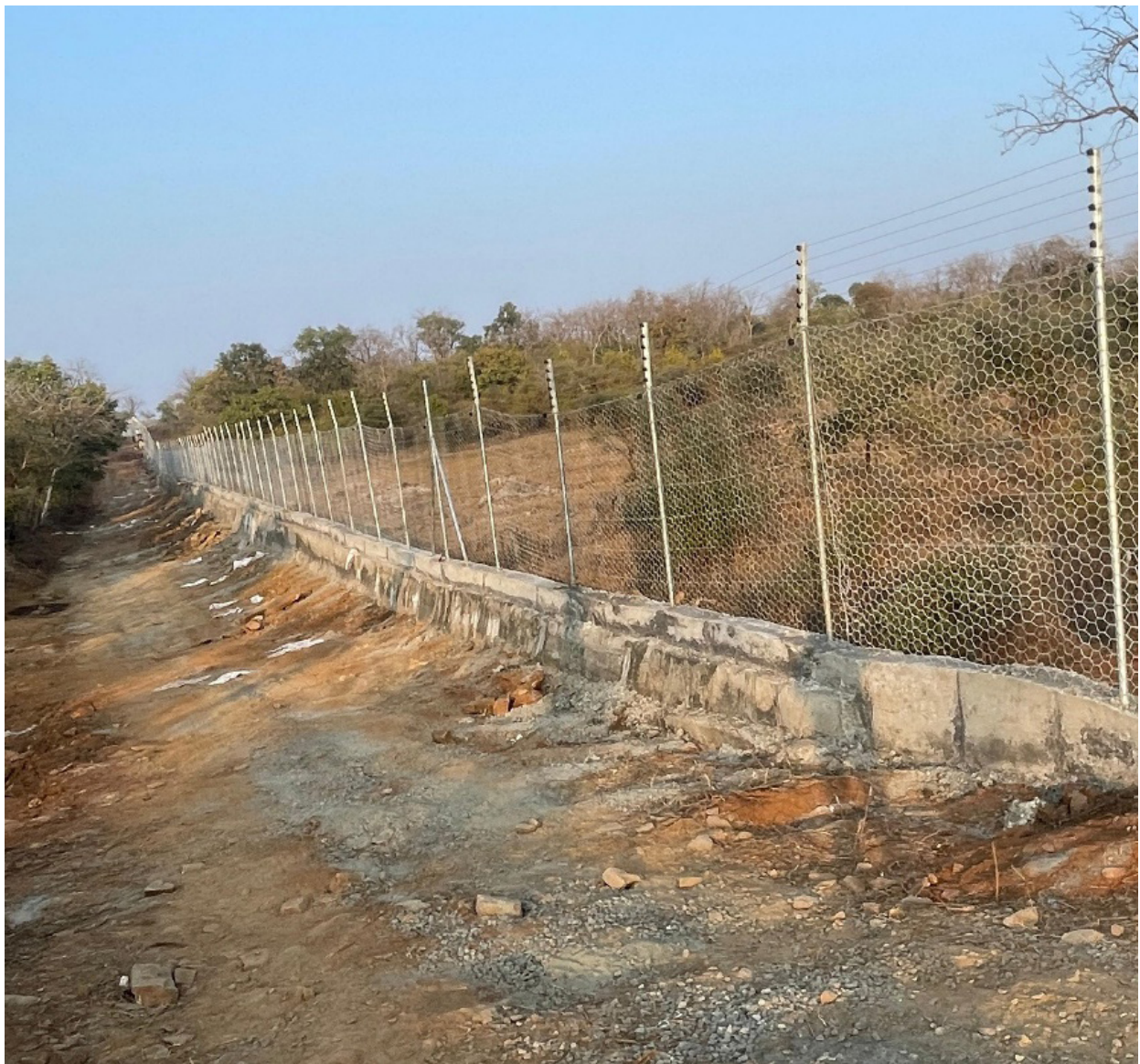
Image 5.4.2. Solar powered predator-proof fence for cheetah release in Gandhi Sagar Wildlife Sanctuary © Madhya Pradesh Forest Department
