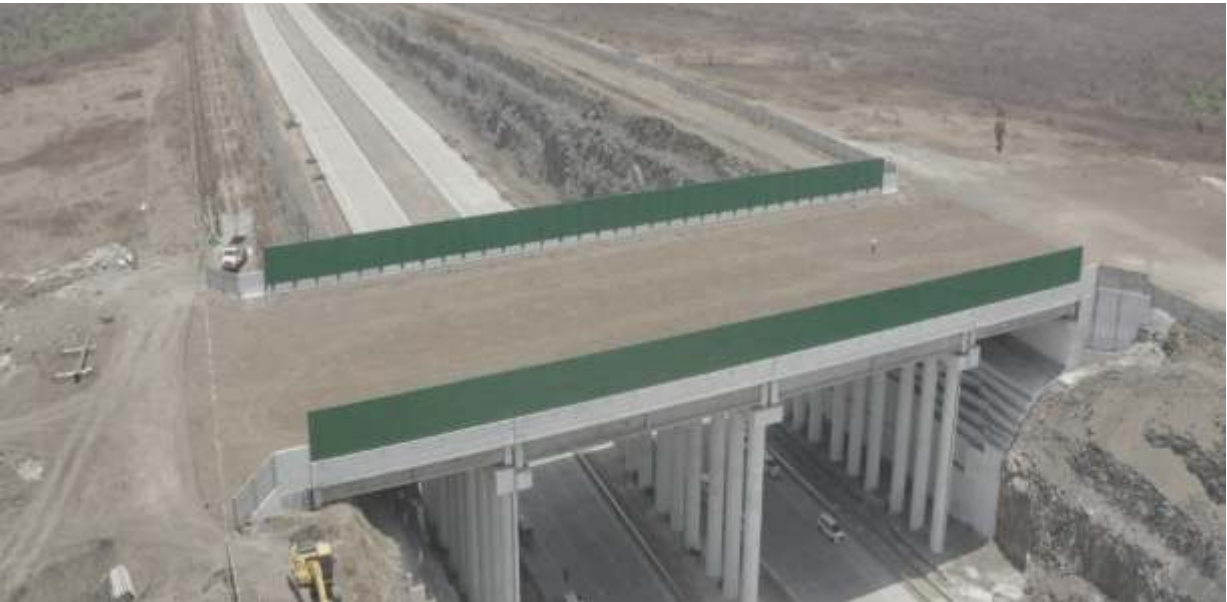
Picture. A wildlife overpass of 60-meter width and 120-meter width is under construction.
